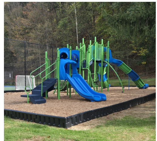
New playground equipment at Ambridge Ave Park
